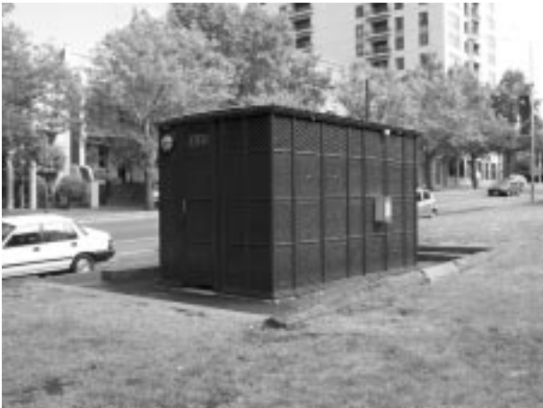
This toilet is located in a highly visible location and provides good opportunity for casual surveillance.
