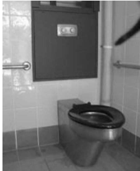
In the above case cistern piping is covered, however the downpipe is vulnerable to vandalism.
